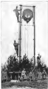
In the picture reproduced above there is shown one of the powerful new searchlights used by the Germans in France. It is built so that it may be telescoped, and carried on a specially constructed wagon
